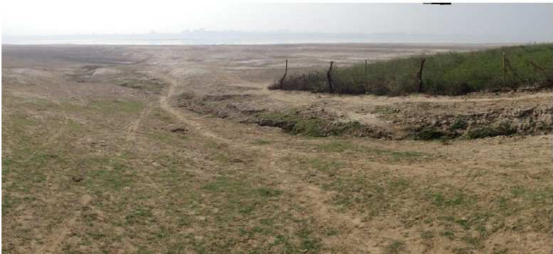
Site Photo: Existing Main Pumping Station at Assi Nallah
