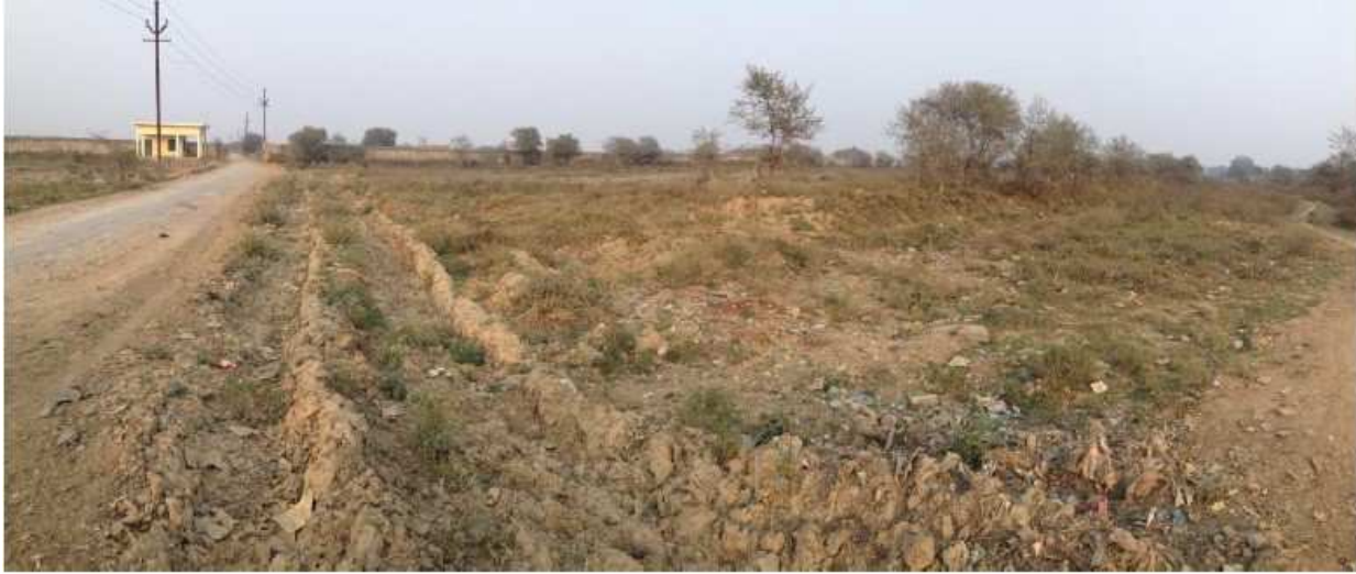
Site Photos: Route of the Effluent Disposal Pipeline
